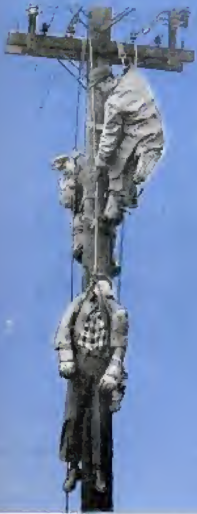
Trouble men of Philadelphia Electric carry out a mock pole-top rescue. Rubber guards placed over line have slipped back, exposing "hot" wire. Worker brushes his head against wire and is knocked unconscious. He falls back against his safety belt and fellow workers rush up pole. One unfastens the victim's safety belt while the other throws a line under his arms and over the crossarm on the pole. Victim is gently lowered to the ground and co-workers administer artificial respiration.
